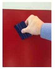
4. Apply the material using firm squeegee strokes. Fix the edges of the corrugation (do not stretch!)
